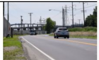
Shown above: Elm Avenue section headed East toward the bridge visible in the background.
