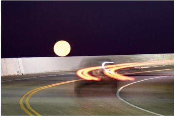
Pictured above: We love the competing elements of this shot by photographer Gregory Hardison that captures a full moon slowly rising behind the bridge with the streaming taillights of a passing vehicle in the foreground.
